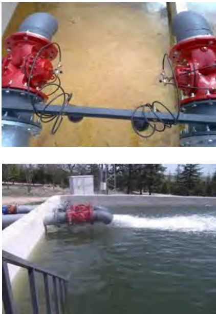
Figure 10. Float valves
