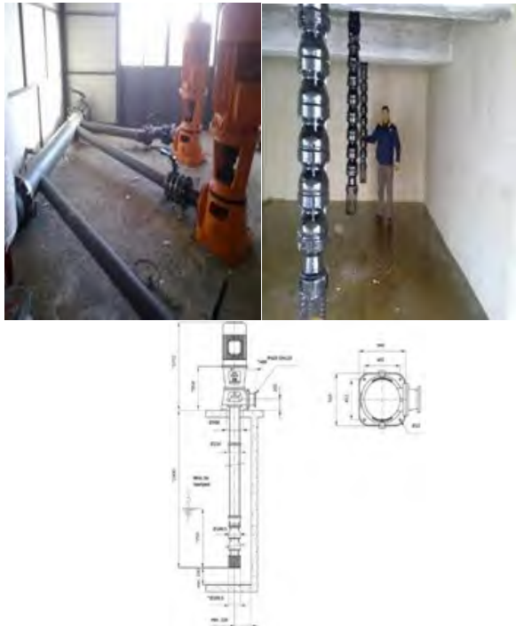
Figure 2. Parallel connected vertical pumps (Polat and Bowler, 2010)
